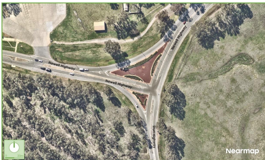
Figure 4: Intersection of Newell Highway and Sturt Highway
