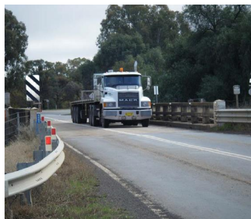
Fig 5: Standard semi-trailer transiting the bridge
