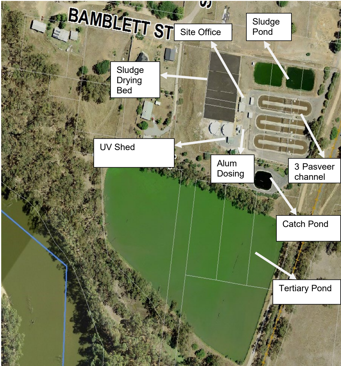
Narrandera Sewer Treatment Plant
