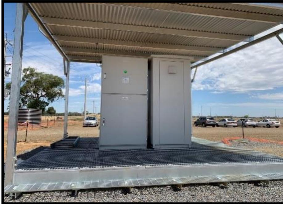
*Figure 18 Typical HV switchboard and platform (Source: ACEnergy)*
