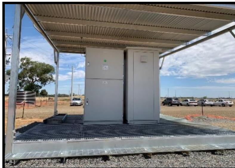
*Figure 19 Typical HV switchboard and platform (Source: ACEnergy)*
