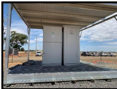
*Figure 15 Typical HV switchboard and platform (Source: ACnergy)*
