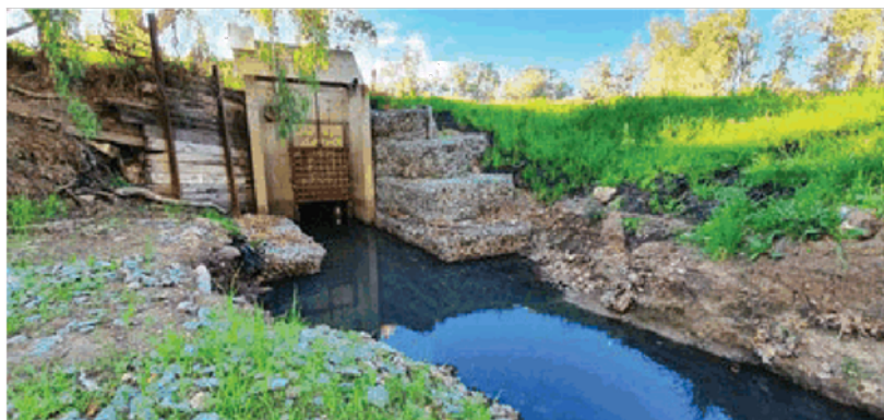
Image: New Gabion Retaining wall replaced failed Siphon Outlet Head wall.
