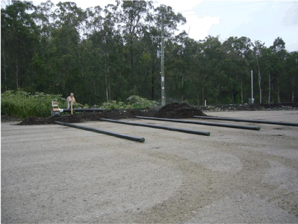
MAF unit laid out and loading commenced
